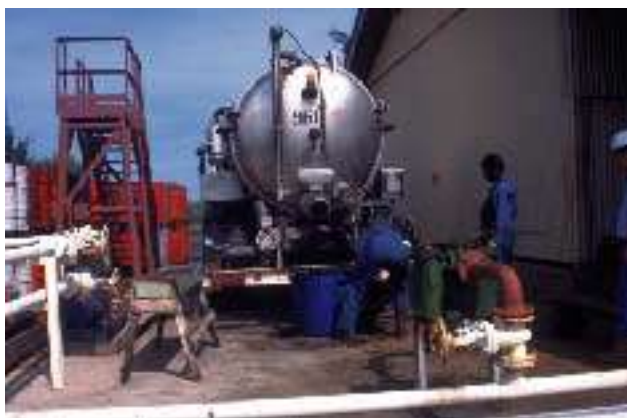
Waste oil is delivered to our plant, then will be weighed out before carrying out a sequence of examination.
